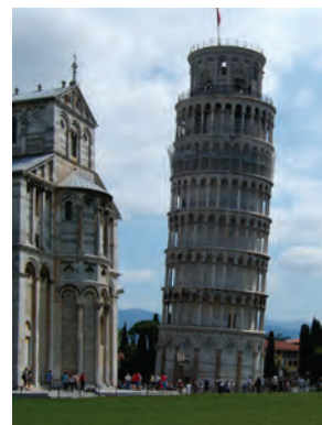
The Leaning Tower of Pisa in Italy was built over a span of 177 years. It began to sink, and lean, while its third floor was being built.
