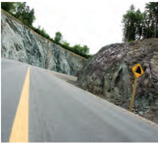
A road's steepness is measured by grade. For example, from Skagway to White Pass, the grade of the South Klondike Highway is 11%.
