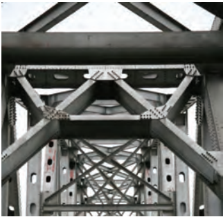
When mitre joints are under pressure or need added stability, gussets are used to reinforce the joint.
