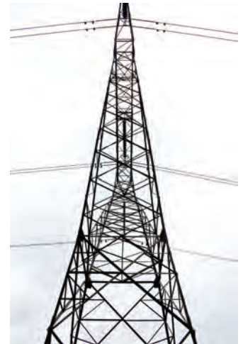
Transmission towers often use a lattice steel pylon design to support cables and conductors.
