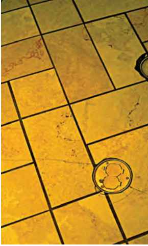
Different-sized tiles are used to set tile in the French pattern.
