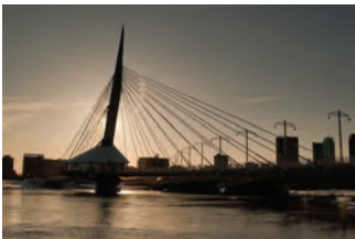
Winnipeg's Esplanade Riel is a side-spar cable-stay bridge designed for pedestrian use. It crosses the Red River to connect downtown Winnipeg with St. Boniface.
