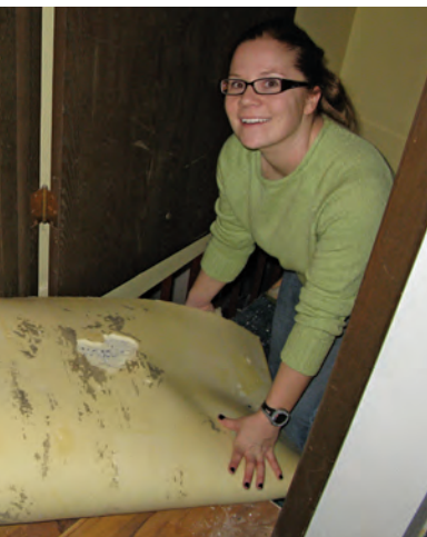
Before installing the new carpet, Giselle removes the old flooring.
