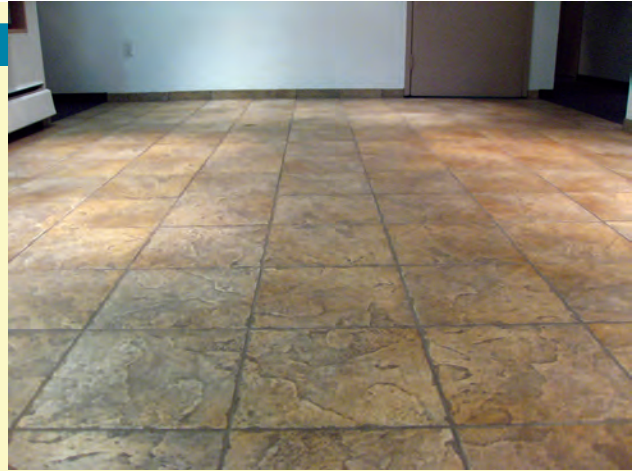
This floor in an apartment building foyer is made of ceramic tiles.
